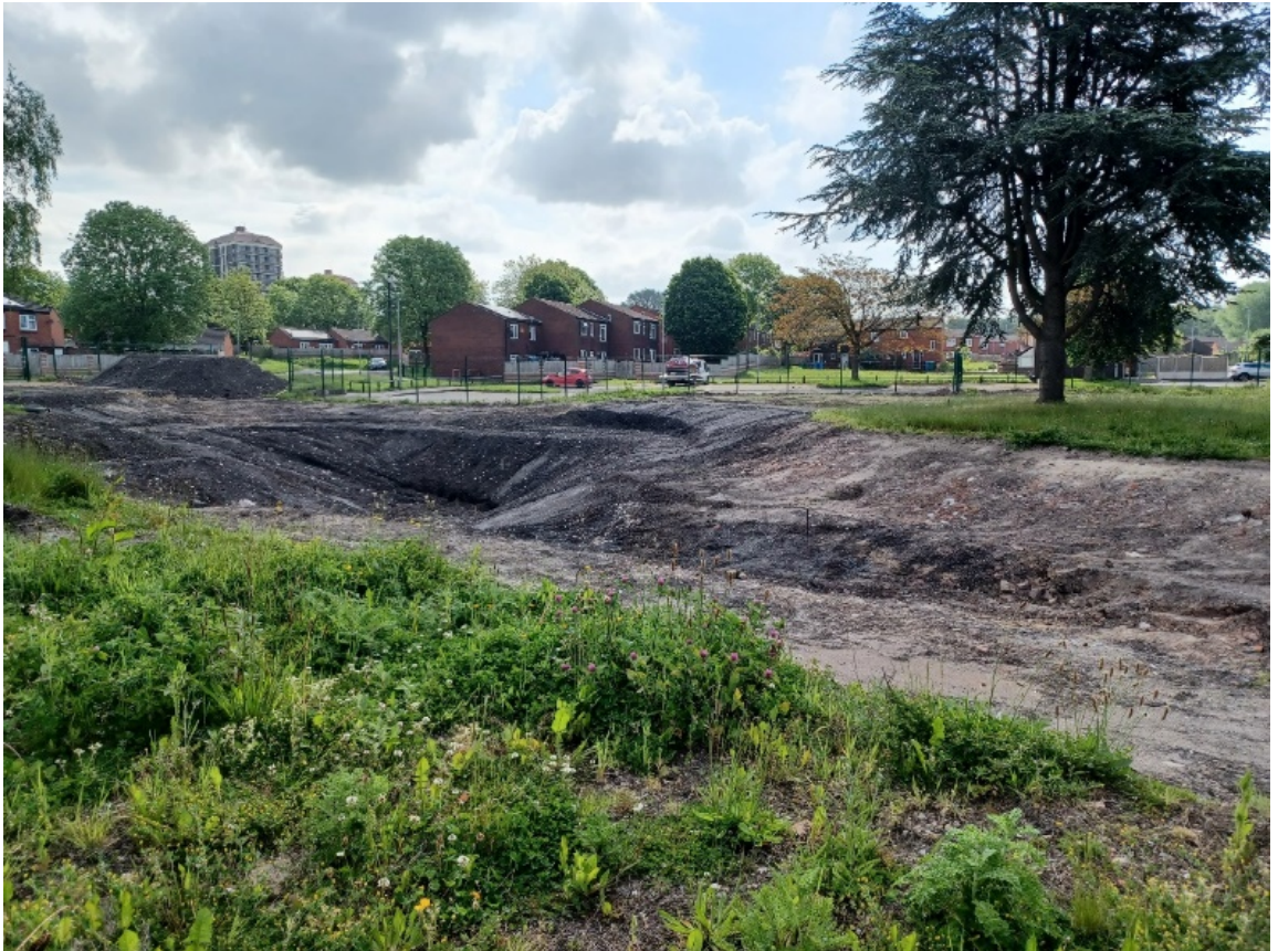
South Collyhurst – Construction of new homes
